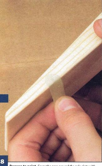
**Prepare to paint.** Cover the area around the axle slots with masking tape to keep paint from filling the slots. Press the tape firmly in place. Paint around the axle slots will cause friction with the wheels and slow your car.
